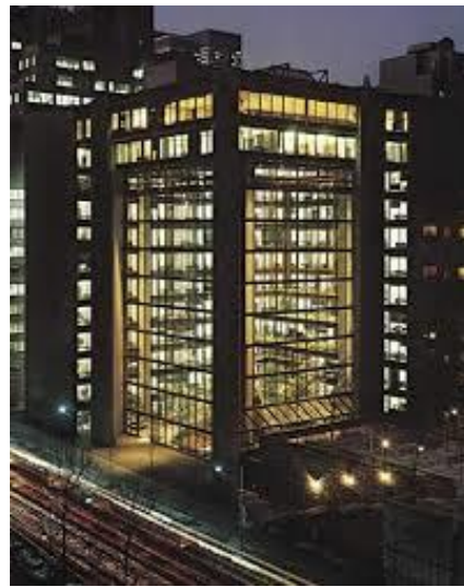
Ford Foundation headquarters. They are green but leave the lights on.
